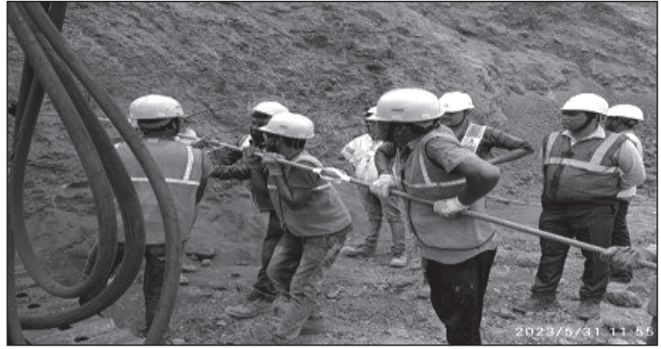
(Figure-02 : Nail installation)
